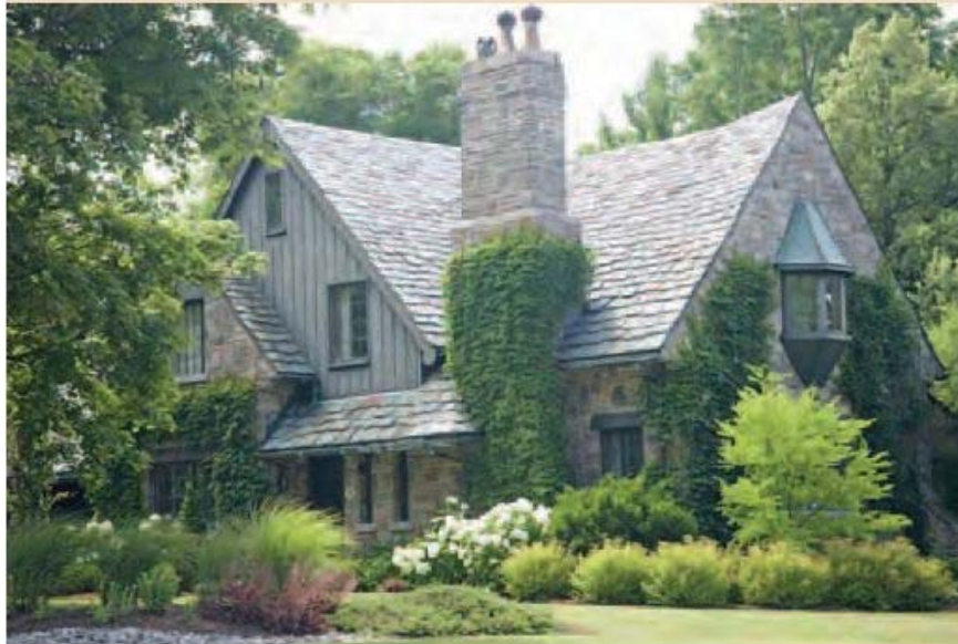
One and One-Half Storey with Stone/Shake Features
